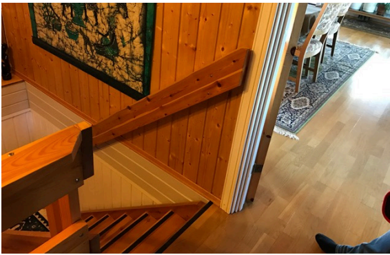
B. Top area of the stair.
