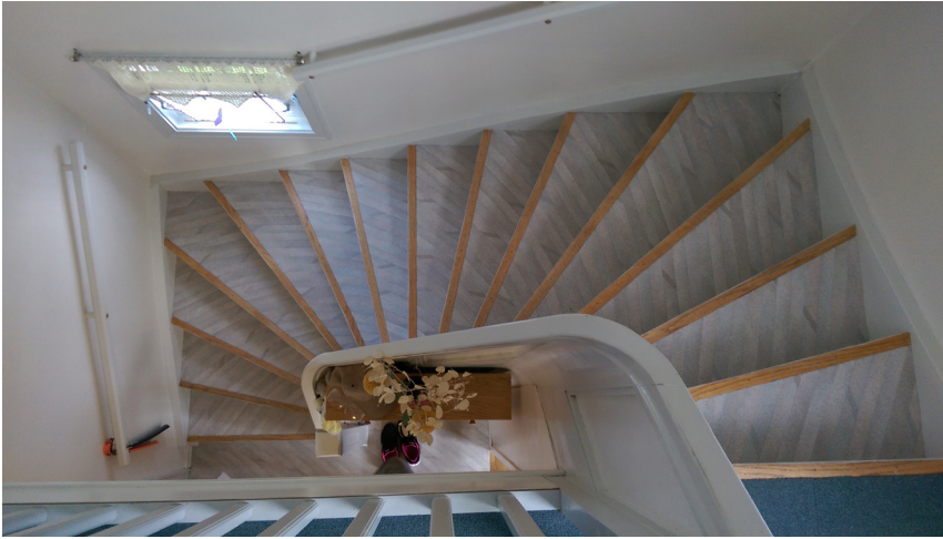
A. Overview pictures showing the whole stair.
