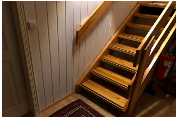
C. Bottom area of the stair.
